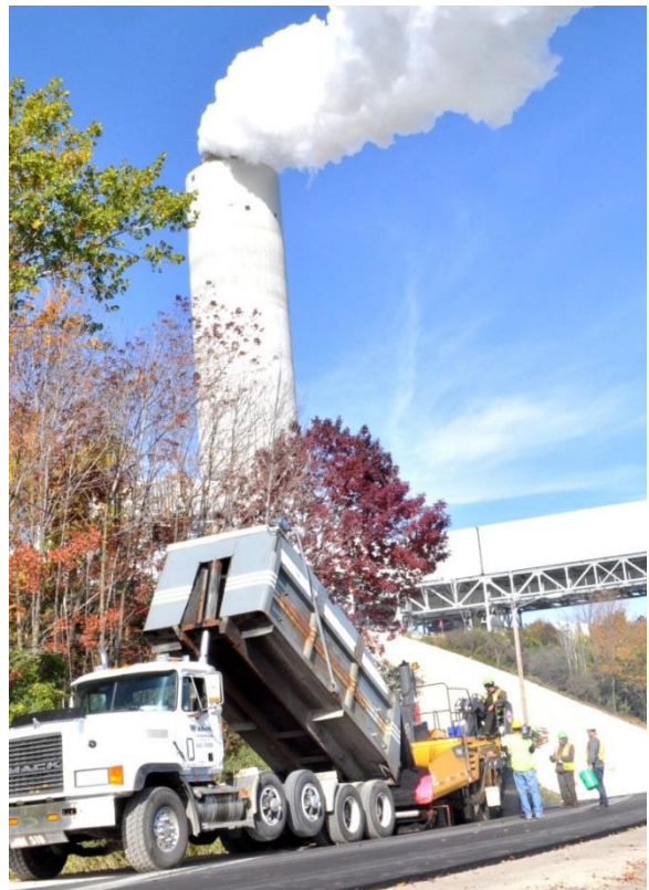
Proof of concept: After lab results pointed to the effectiveness of using fly ash as an ingredient in asphalt, We Energies field-tested ASHphalt by using it to pave a road at its Oak Creek coal plant.
