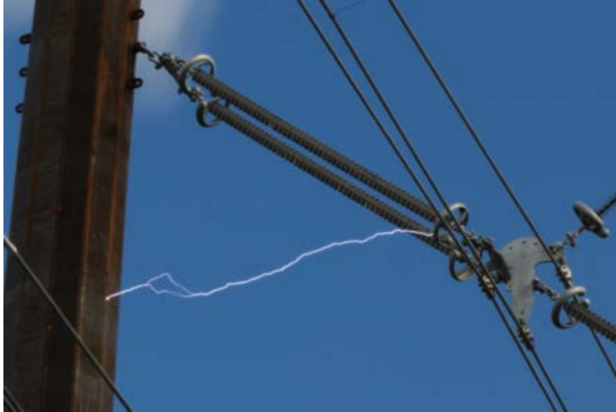
Lightning tests on a BOLD line. Photo taken as part of AEP testing performed at EPRI's Lenox, Massachusetts laboratory.
