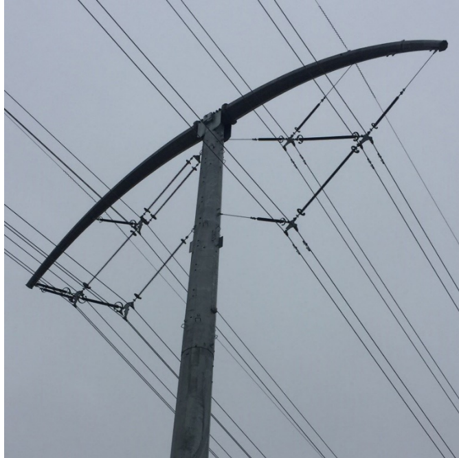
AEP's first 345-kilovolt BOLD line in Indiana. Conductors are suspended from a crescent-shaped crossarm on a 100-foot tubular steel pole.
