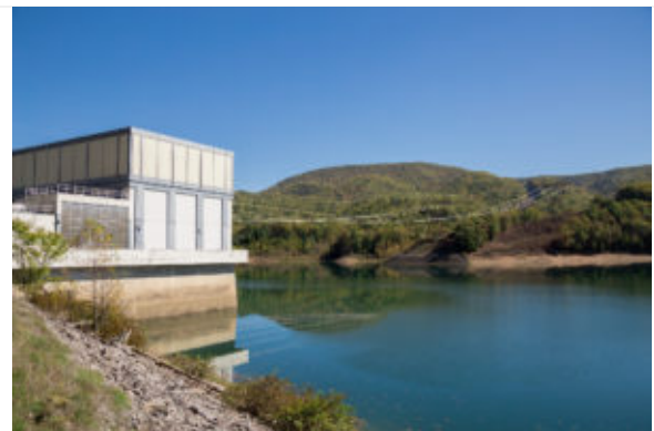
The Bath County Pumped Storage Station in Virginia's Allegheny Mountains has a capacity of more than 3,000 megawatts. Photo courtesy of Jeffrey G. Ocampo, Dominion Energy.
