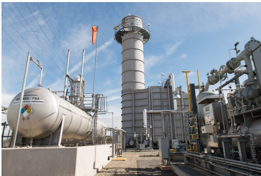
In 2017, Southern California Edison deployed this hybrid natural gas turbine/battery energy storage system. The 10-megawatt battery system enables the gas plant to respond more quickly to changing grid needs. Photo courtesy of Edison International.
