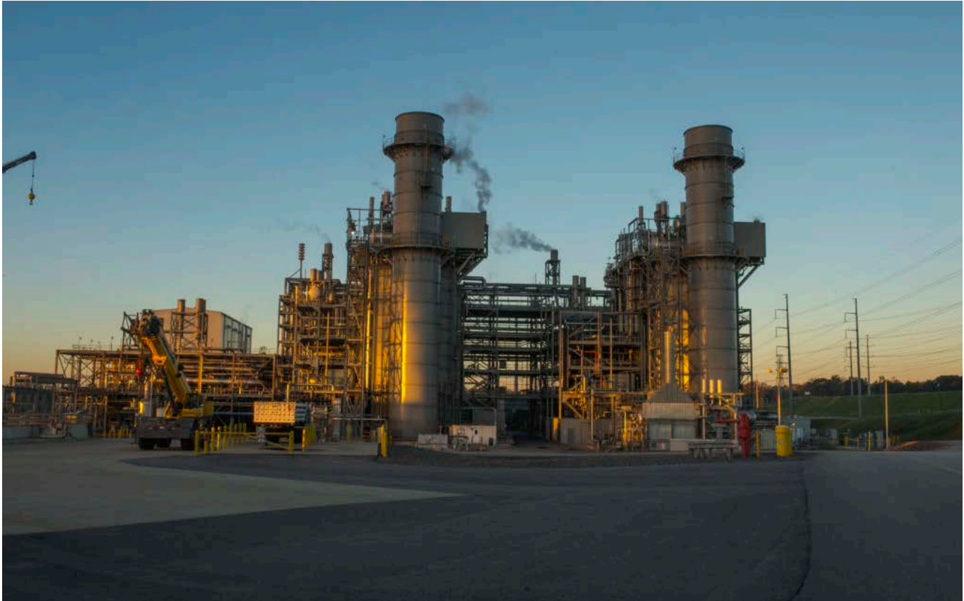
Georgia Power's Plant McDonough-Atkinson. Photo courtesy of Georgia Power. [click to enlarge]
