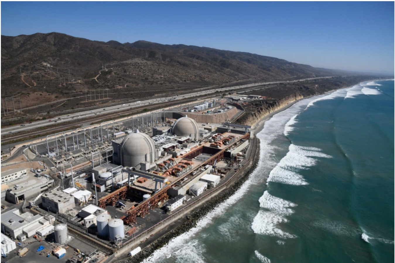
In-plane fluid elastic instability was observed for the first time in an operating steam generator in 2012 at San Onofre Nuclear Generating Station in California. Photo courtesy of Southern California Edison.
