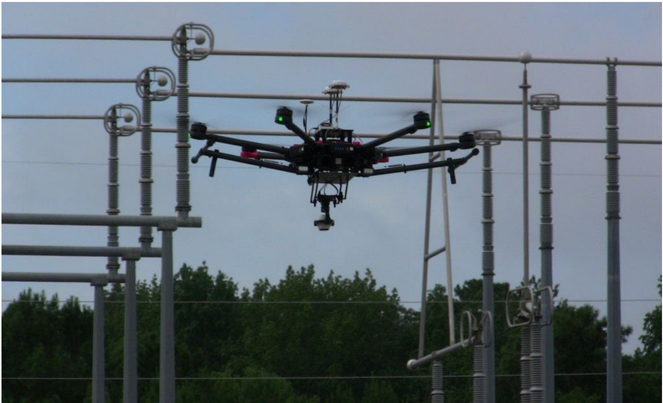
A drone collecting images of substation equipment during an EPRI field test.
