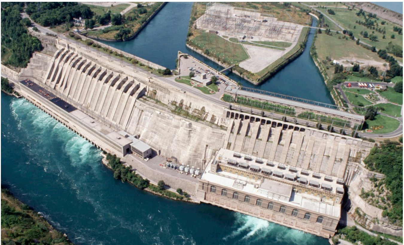
Sir Adam Beck Generating Station, a hydropower facility in Queenston, Ontario. Photo courtesy of OPG.
